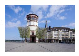
building is newly coated with the systone sol silicate with a mineral facade colour, which is compatible with the non-mineral old coating, presenting a bright exterior tone, endowing the historic tower building with a new look once again.
